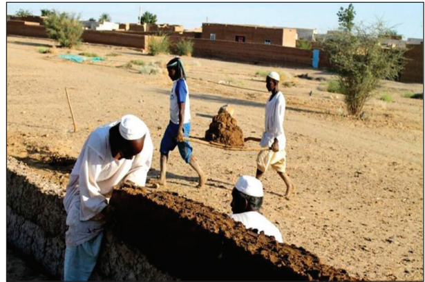
Fig. 15a: Part of the 4.2 km mud wall protecting the site .
